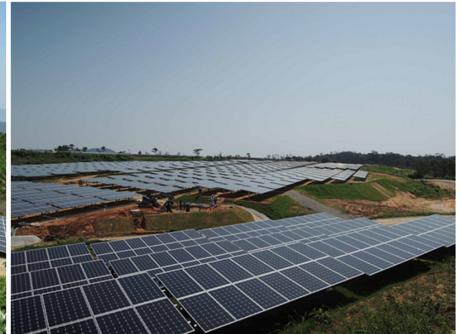
Ichigo Nago Futami ECO Power Plant (Okinawa)
